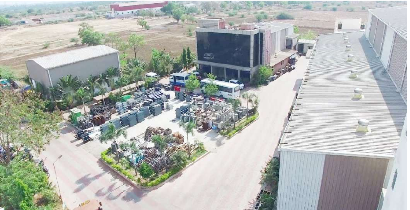
Voltech Techno Park - III Power & Distribution Transformers Manufacturing Facility
