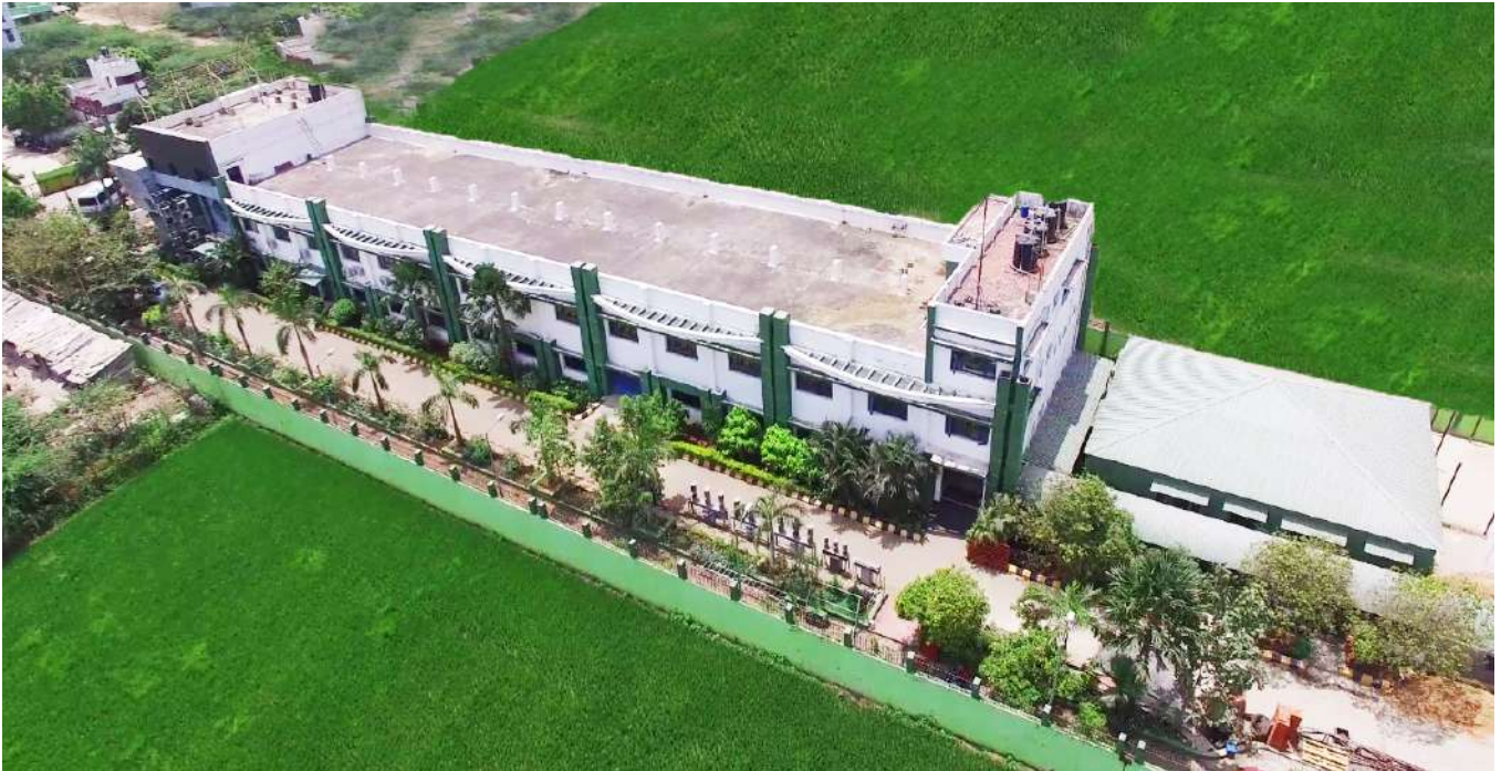
Voltech Techno Park - I Relays, Electronics & Solar Manufacturing Facility
