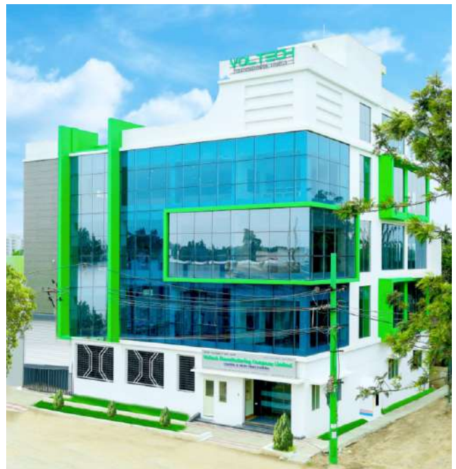
Voltech Techno Park - IV Control & Relay Panel Manufacturing Facility
